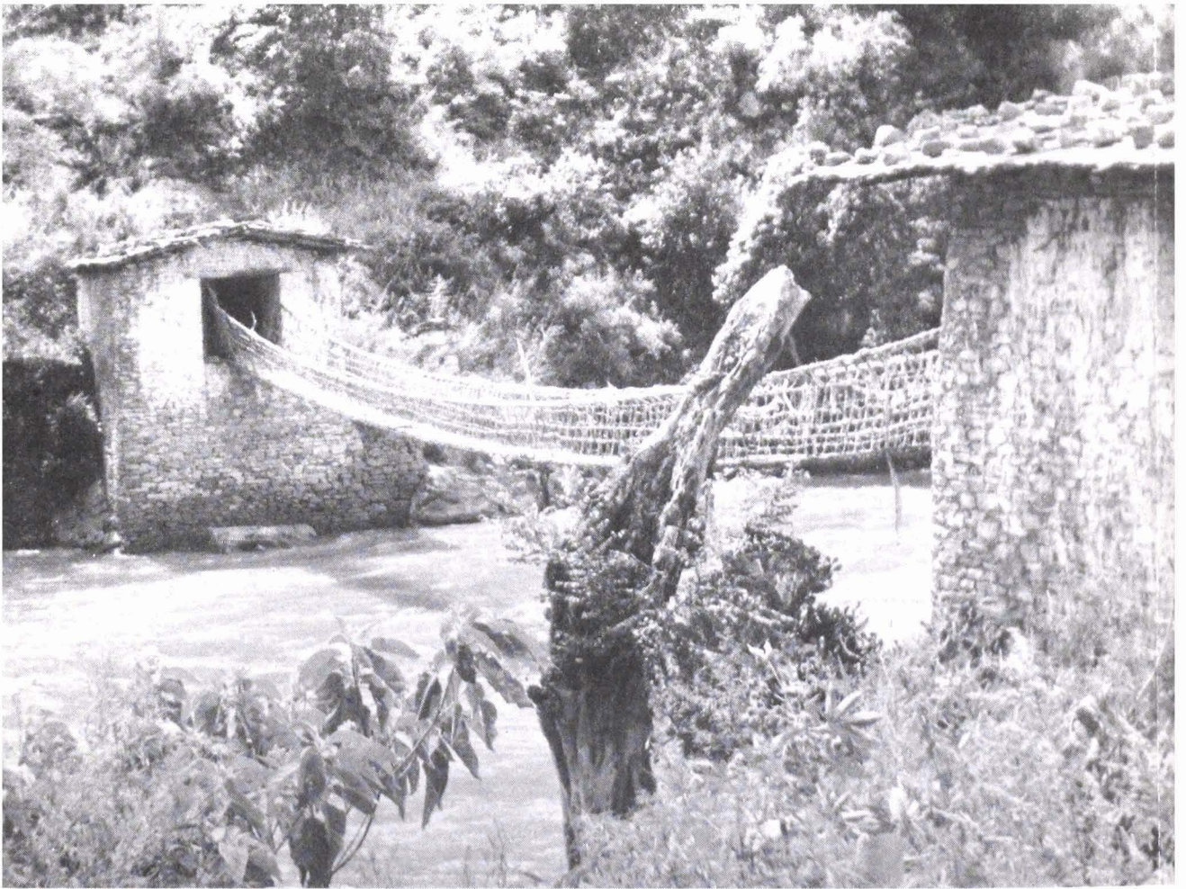
Ropes of twisted bamboo support countless bridges in Bhutan. There was a near disaster when two mules tried to cross the lower one, at Lhuntse, at the same moment
